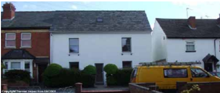
Simmonds.Mills / Thermal Inspections Ltd
